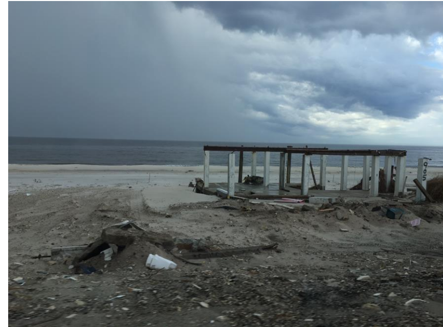
Aftermath of Hurricane Michael damage along Gulf of Mexico
